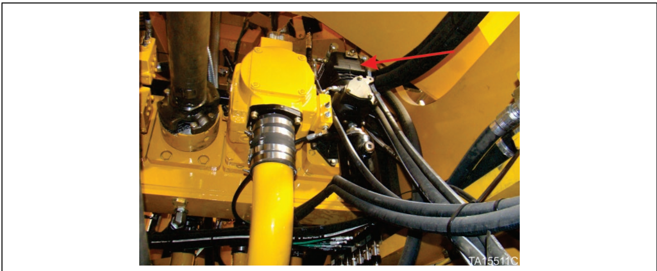
Figure 2. Air compressor location (gearbox-Hydraulic Pump Drive (HPD) mounted)
